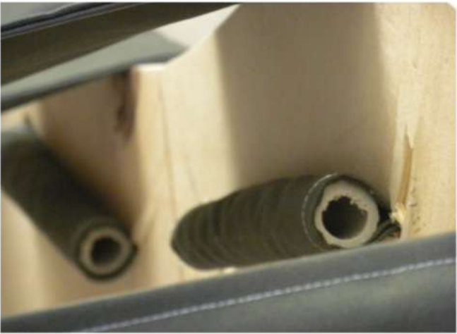
PVC pipe was used to hook in the fabric straps into the wooden slots.
